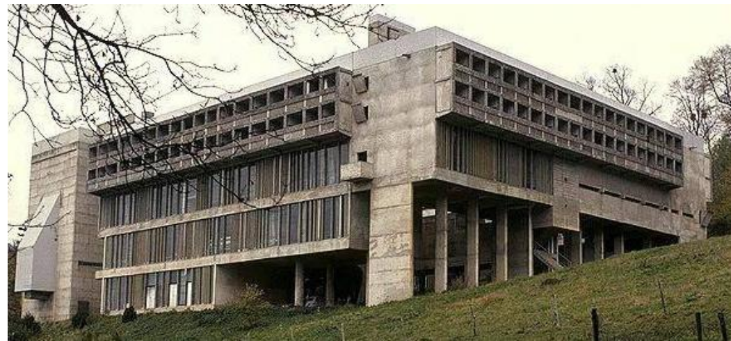
La Tourette monastery, France (1957-60)
